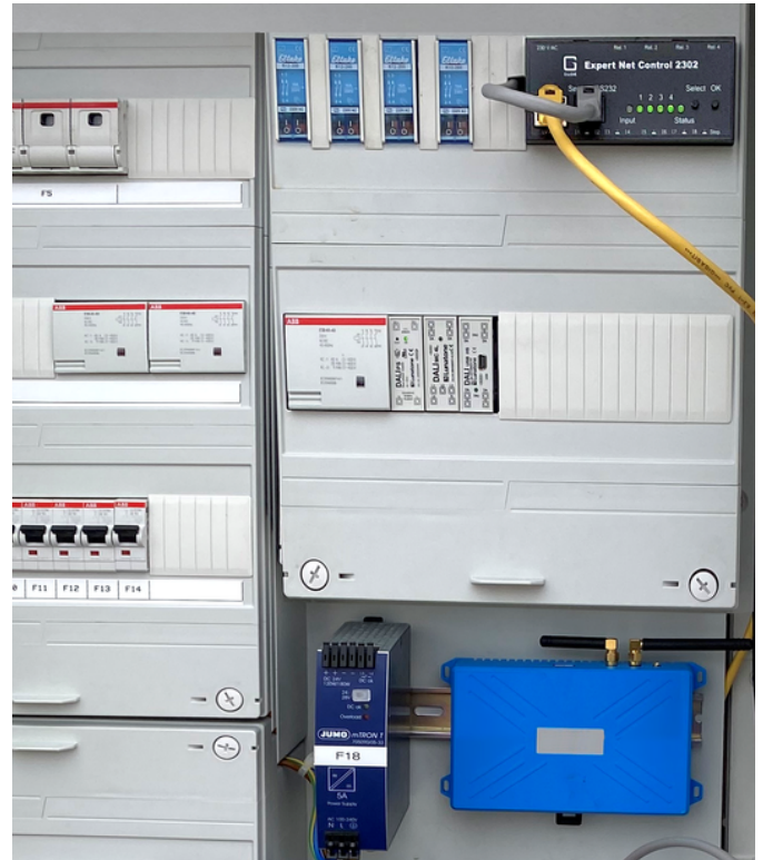
Expert Net Control 2302 in the switch cabinet (upper right), Photo: City of Monheim
